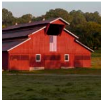
Hillsboro Barn Franklin, TN
